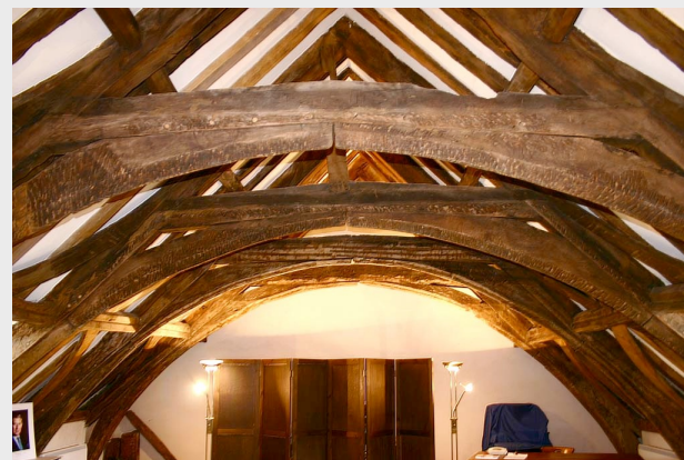
The roof of 21 The Mint
