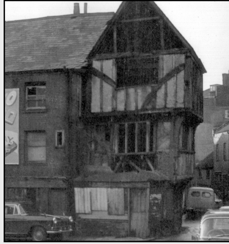
The house before the move
