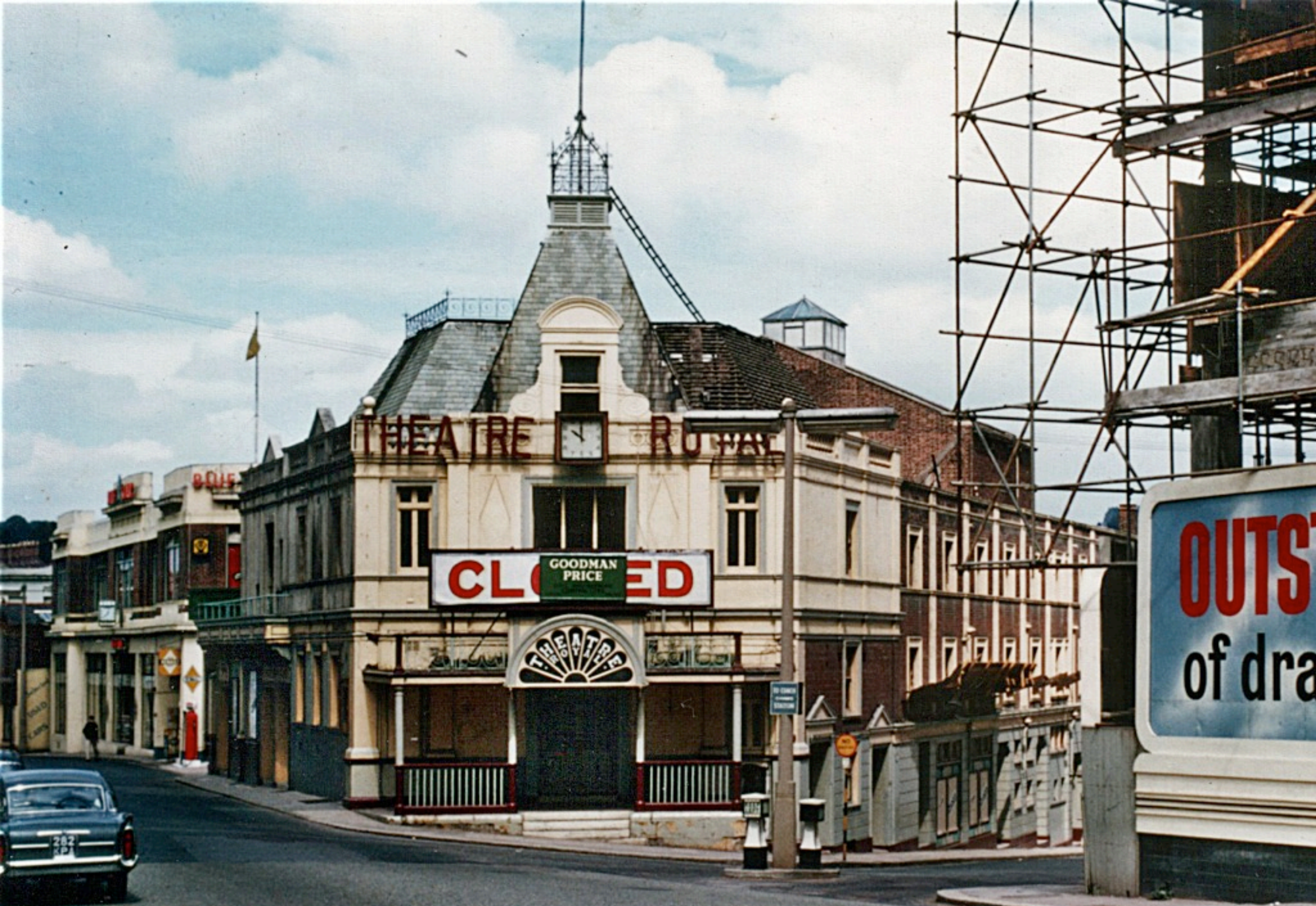
The forlorn Theatre Royal awaits demolition, as a new store is constructed opposite –1962
